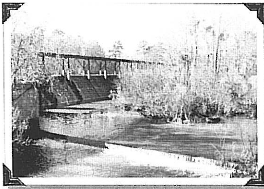
The Long-gate Spillway is one of the many significant structures along the Canal surveyed by the Historic American Engineering Record.
